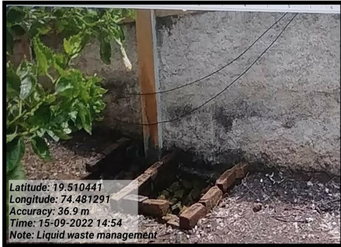
Liquid Waste Management System (Soak pits)
