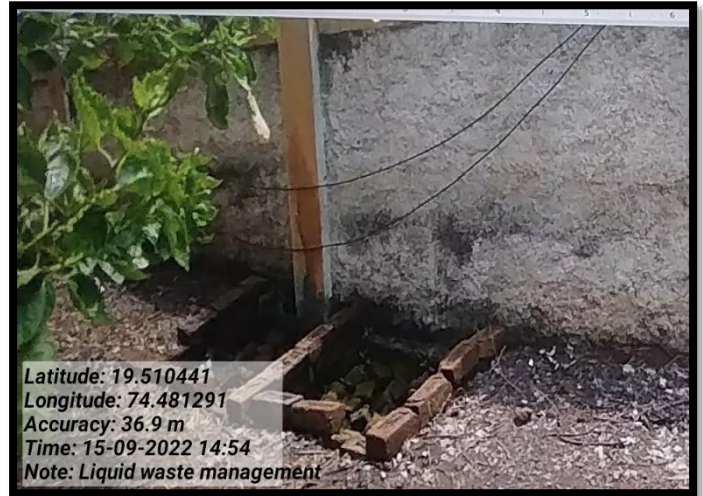
Liquid Waste Management System (Soak pits)
