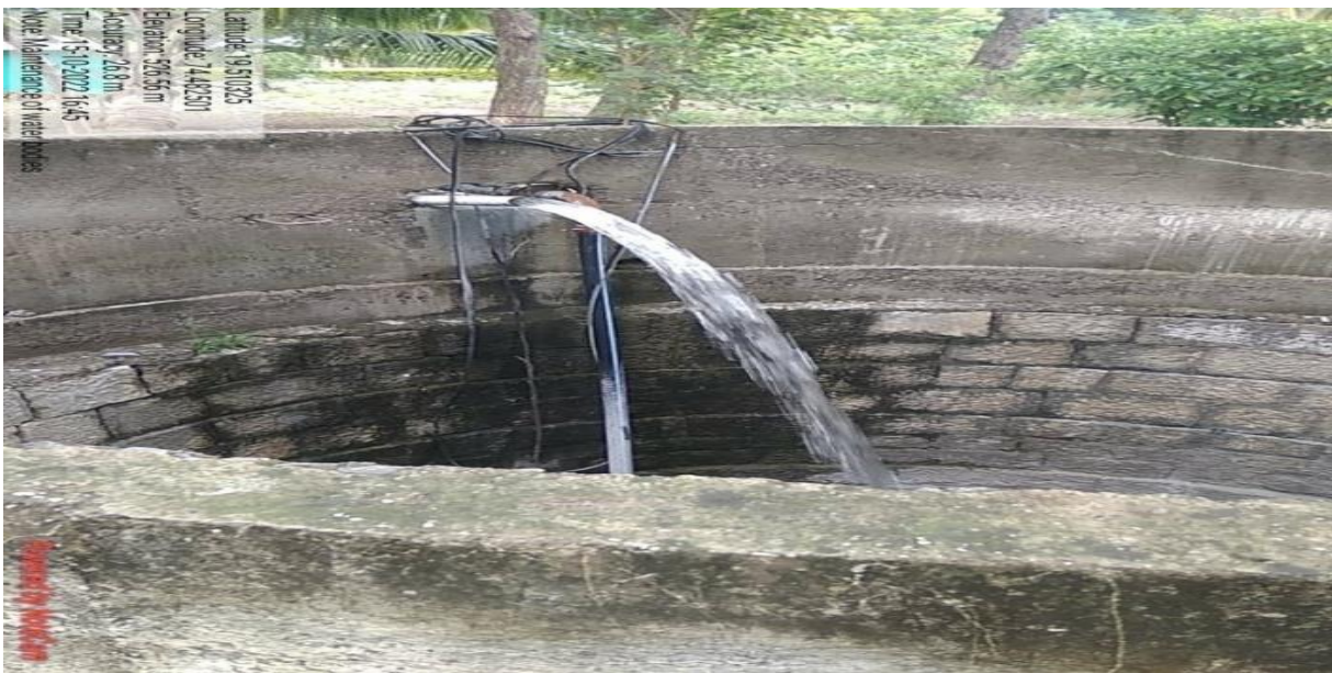
Photo:Rain Water Harvesting Date:15/10/2022
