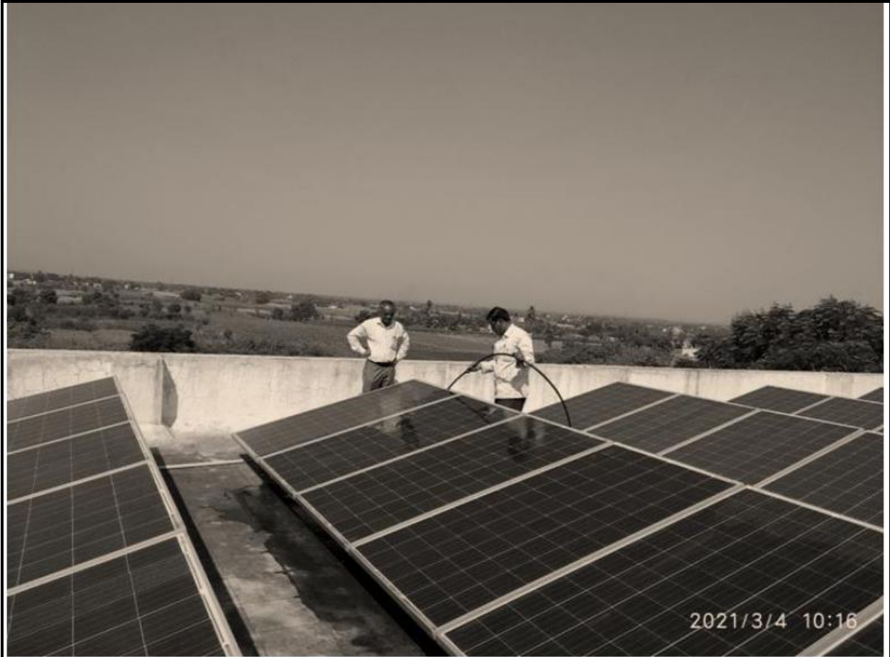
Figure: Mr. Rajdeo B. U. Demonstrating enhanced efficiency after cleaning the solar panel in virtual mode
