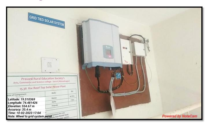
**Solar Energy Wheel to Grid System Panel**
