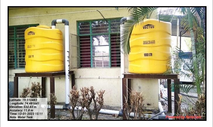
Water Tank for collection of Rain Water Harvesting
